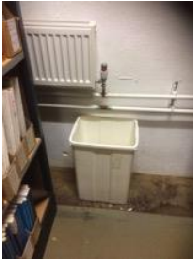
Image 3: Leaking radiator
